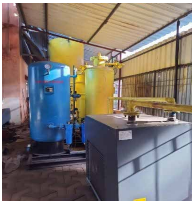
Figure 2: Pilot scale Nitrogen generator
