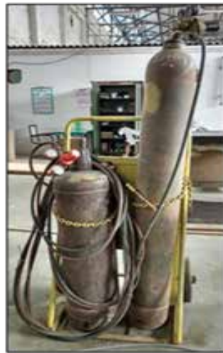
GAS WELDING PLANT
